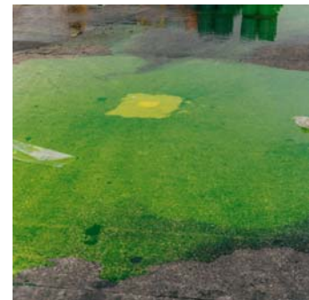
Demonstration of a clay drain mat in use preventing coloured water entering a drain.
