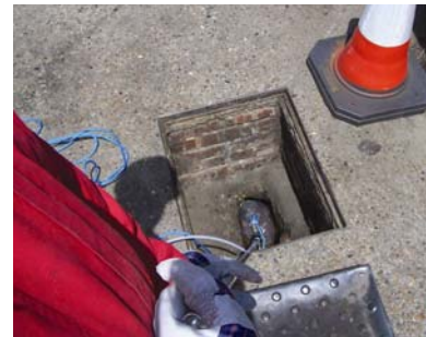
A pipe blocker being inserted into a drain.
