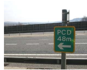
Sign indicating location of a highway pollution control device (PCD). Photo credit: Highways Agency
